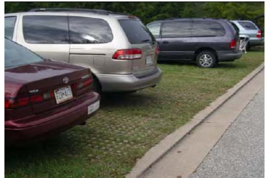
Parking area with permeable pavers
