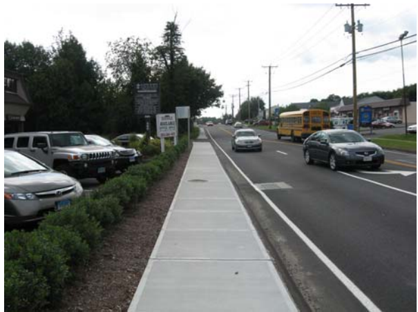
New sidewalks along Route 111
