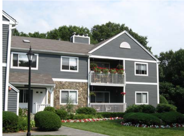
Typical multi-family units in The Hills of Monroe development
