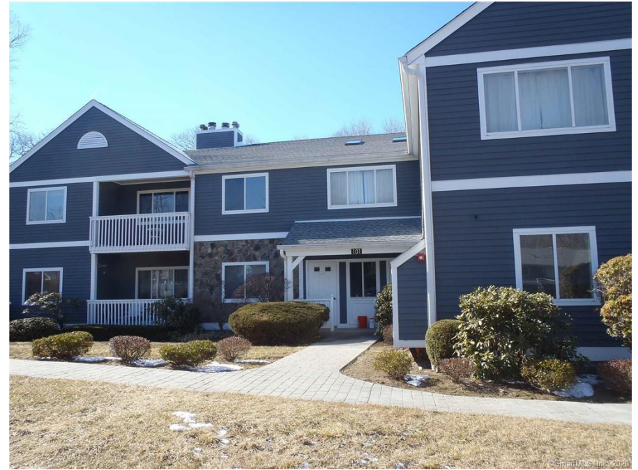
Non single-family detached housing, such as The Hills of Monroe, comprises less than 15% of housing stock in Monroe. Image Source: Coldwell Banker
