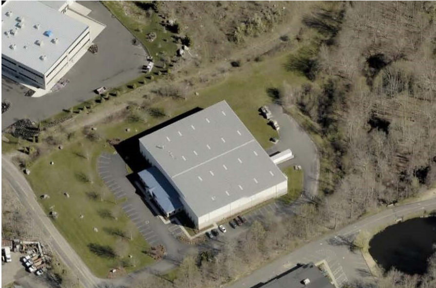
Pepper Street Industrial Park, Image Source: Loopnet.com
