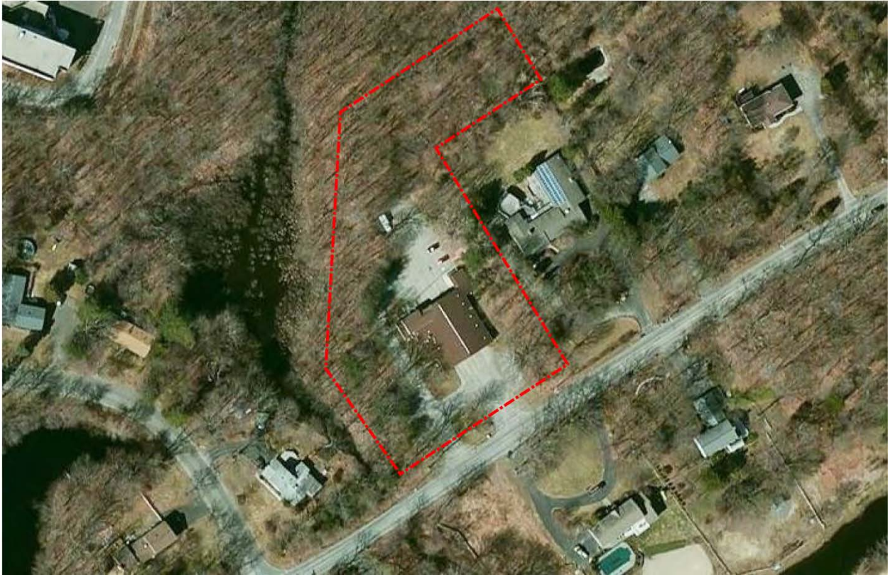
Aerial View showing Extents of Property
