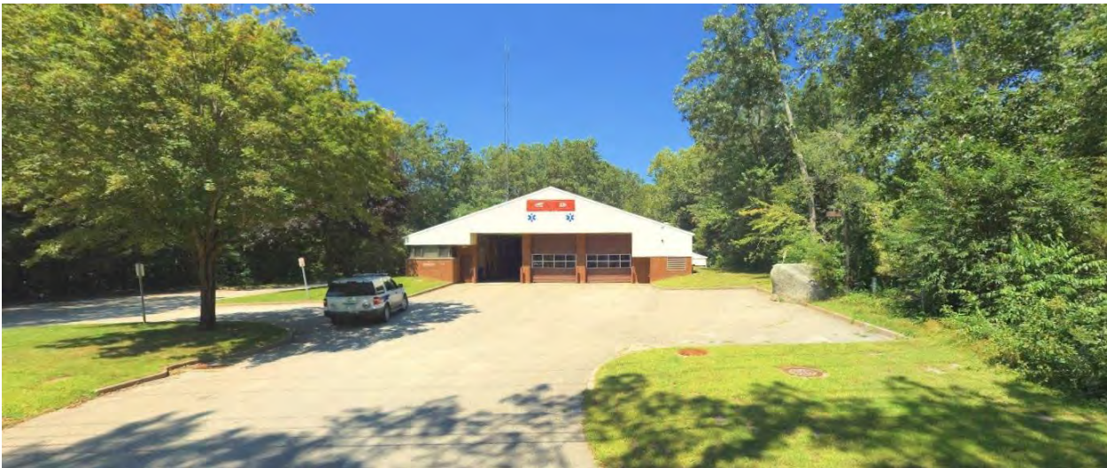
View of 54 Jockey Hollow Road from street looking north
